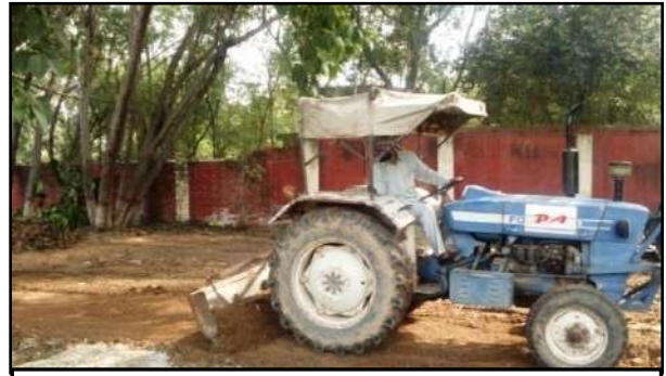
Leveling of the stretch
