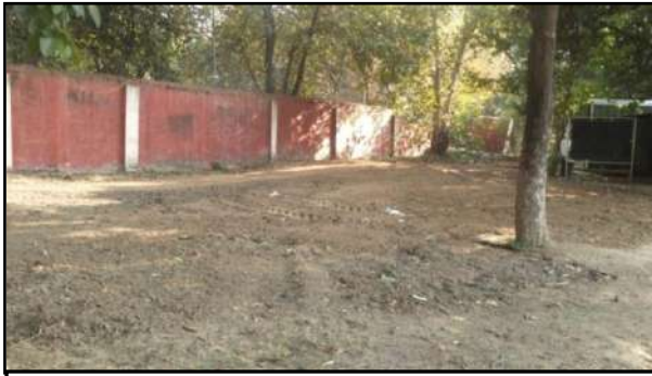
Land after initial digging
