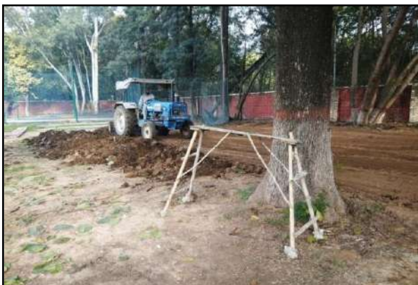
Leveling of the stretch
