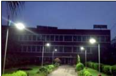
Solar Lights in college campus
