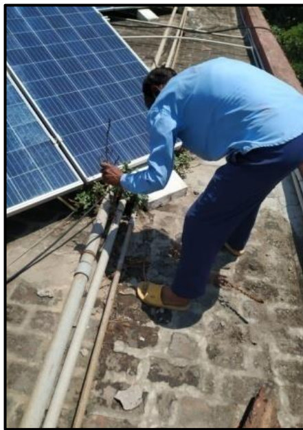
Cleaning of the roof top tanks, underground water tanks, roof area and water coolers
