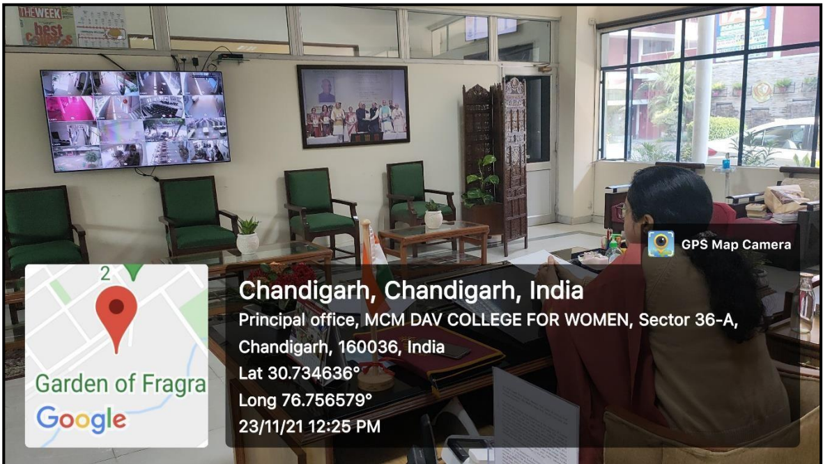
DVR Units and Screen Monitor for CCTV surveillance in Principal office
