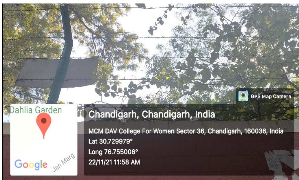
Barbed Wires on High Boundary Walls
