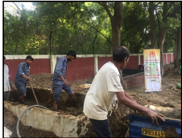
Addition of Cow dung to Initiate the Production of Biogas
