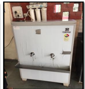
Sample-5 ; Water Cooler; Near E Block Mess
