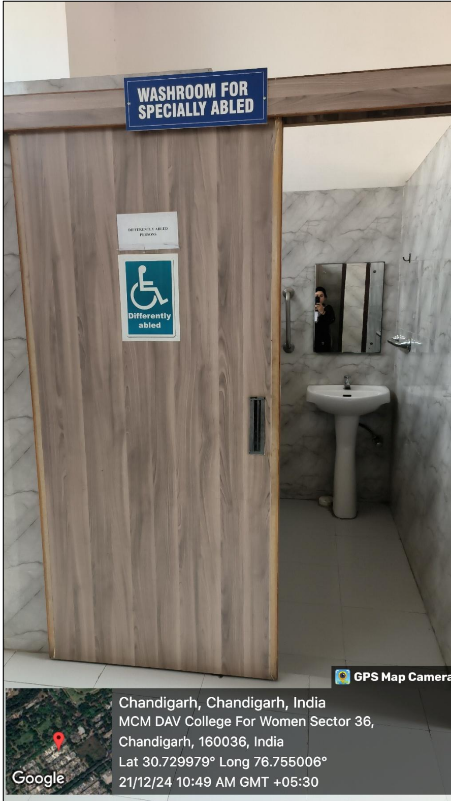
Washrooms for Specially abled persons
